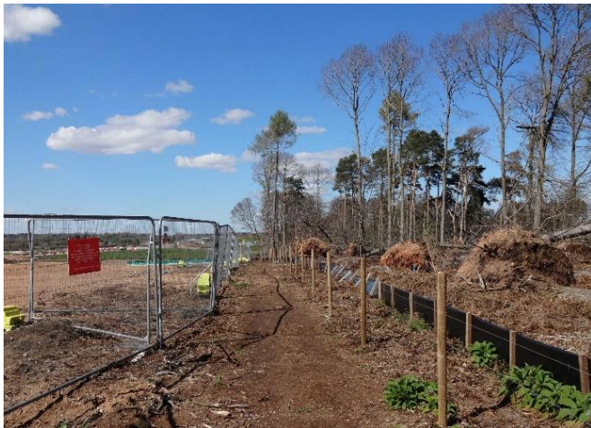
HS2 works between Meriden and Barston
