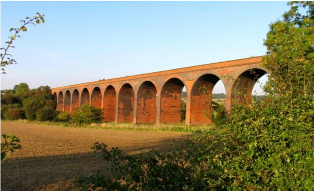
John O'Gaunt viaduct, north of the Marefield Triangle on the LNWR trackbed. © Andrew Tatlow (cc-by-sa/2.0).
