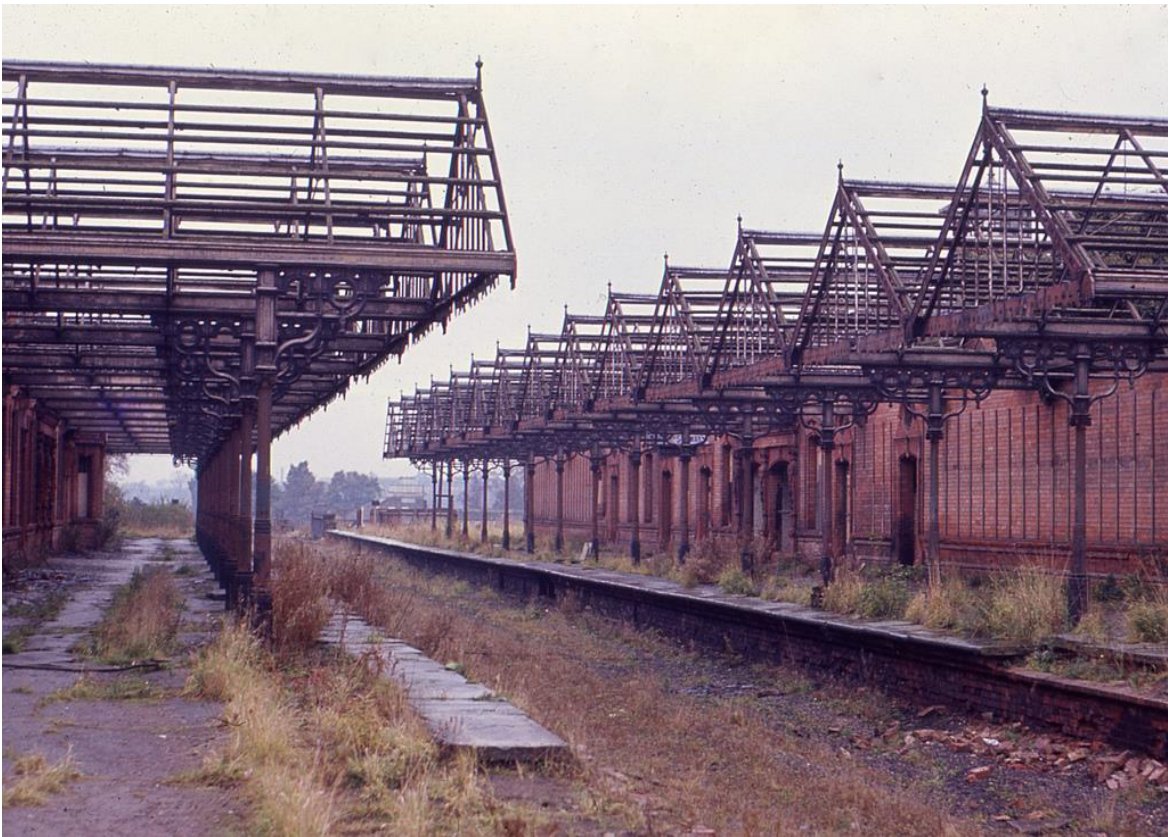
The sad sight of Melton Mowbray North Station in the process of being demolished. Photograph by John Evans.
