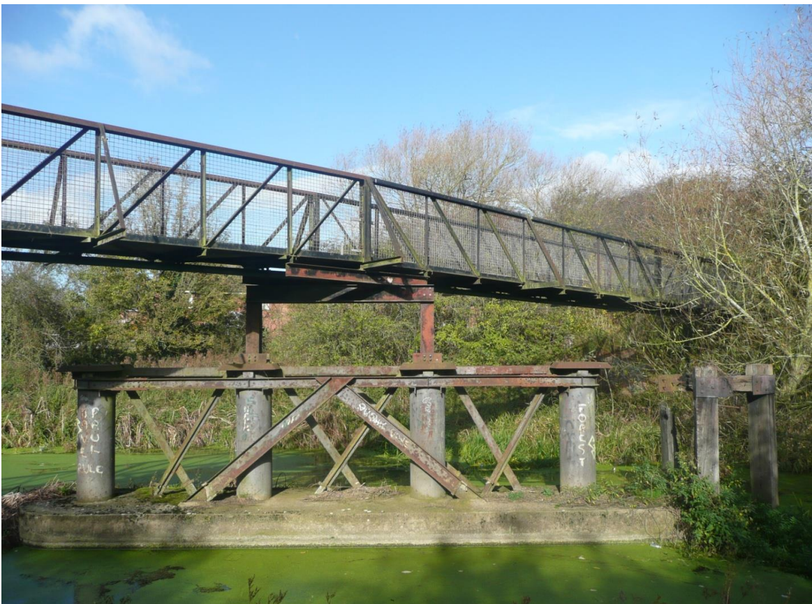
Two views of the support for the original bridge over the River Eye of the LNWR, en route to Melton Mowbray North Station, which was demolished following total closure of the line in 1964 – the site is now a retail estate. What we see here is a footbridge grafted on to the original supports; an incongruous looking, Heath Robinson type, affair.
