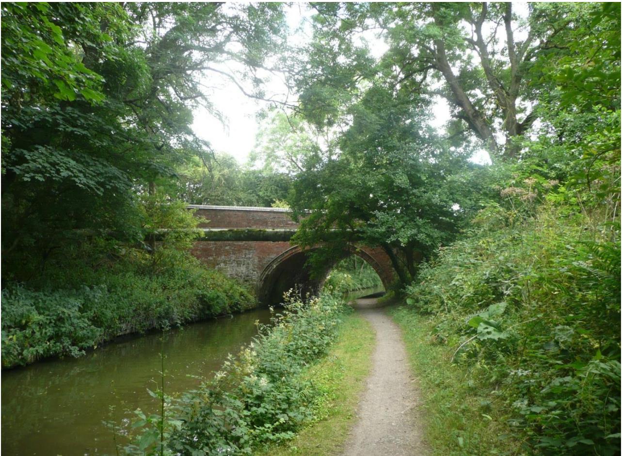
The Grand Union Canal, Market Harborough arm, at Gallows Bridge (no. 8) at the B6047. It was a humid day in July 2017. The pipe crossing the canal in front of the bridge belongs to the factory which is out of shot behind the hedge on the right. Our route along part of The Leicestershire Round passes through the factory precincts.
