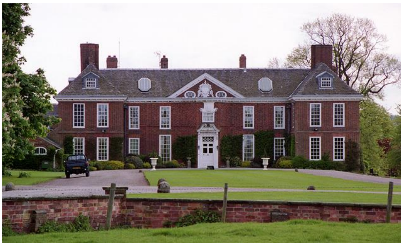
Lowesby Hall, front elevation, as seen from the grassed footpath described in our Directions. © Stephen Richards (cc-by-sa/2.0).
