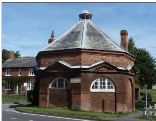
Fig. 1.5 The unusual Church Hall at Burwell
